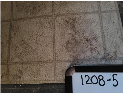
1208-5 12"x12" Floor Tile/Adhesive Interior Bathroom
