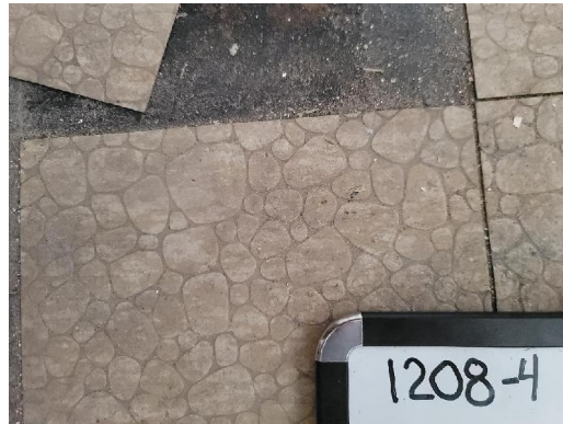
1208-4 9'x9" Floor Tile/Beige (3% Chrysotile) Mastic/Black (3% Chrysotile) Typical Interior (Appx. 492 sq feet)
