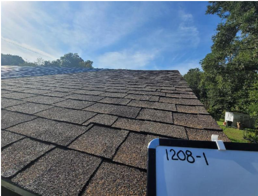
1208-1 Asphalt Shingle/Tar Typical Exterior Roof
