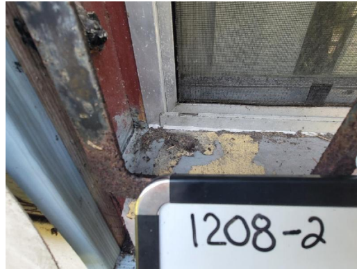
1208-2 Caulk Typical Exterior Windows
